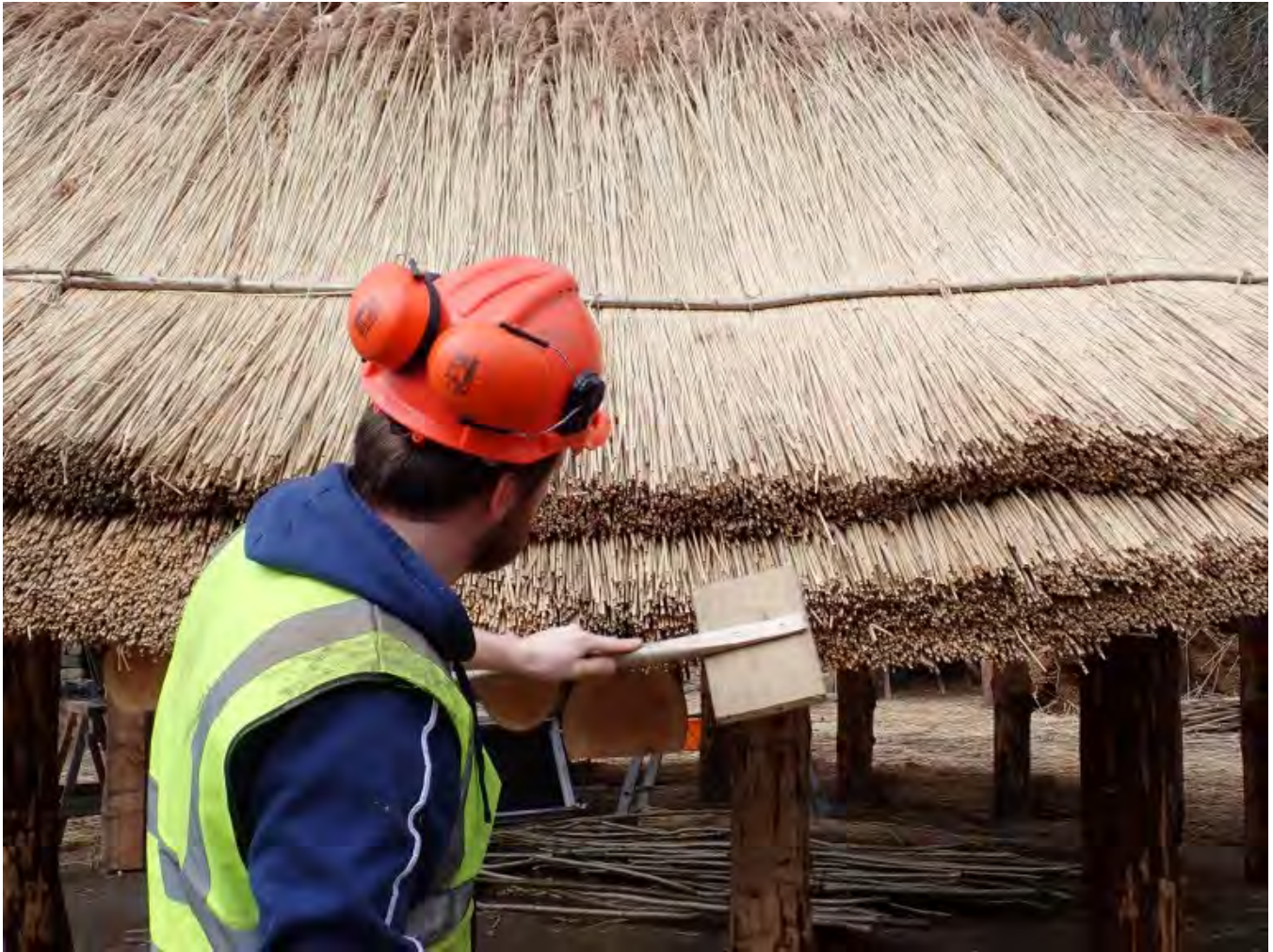
Fig 25. Ross, Vernacular Buildings Craft Fellow, working on thatch at the Scottish Crannog Centre.
