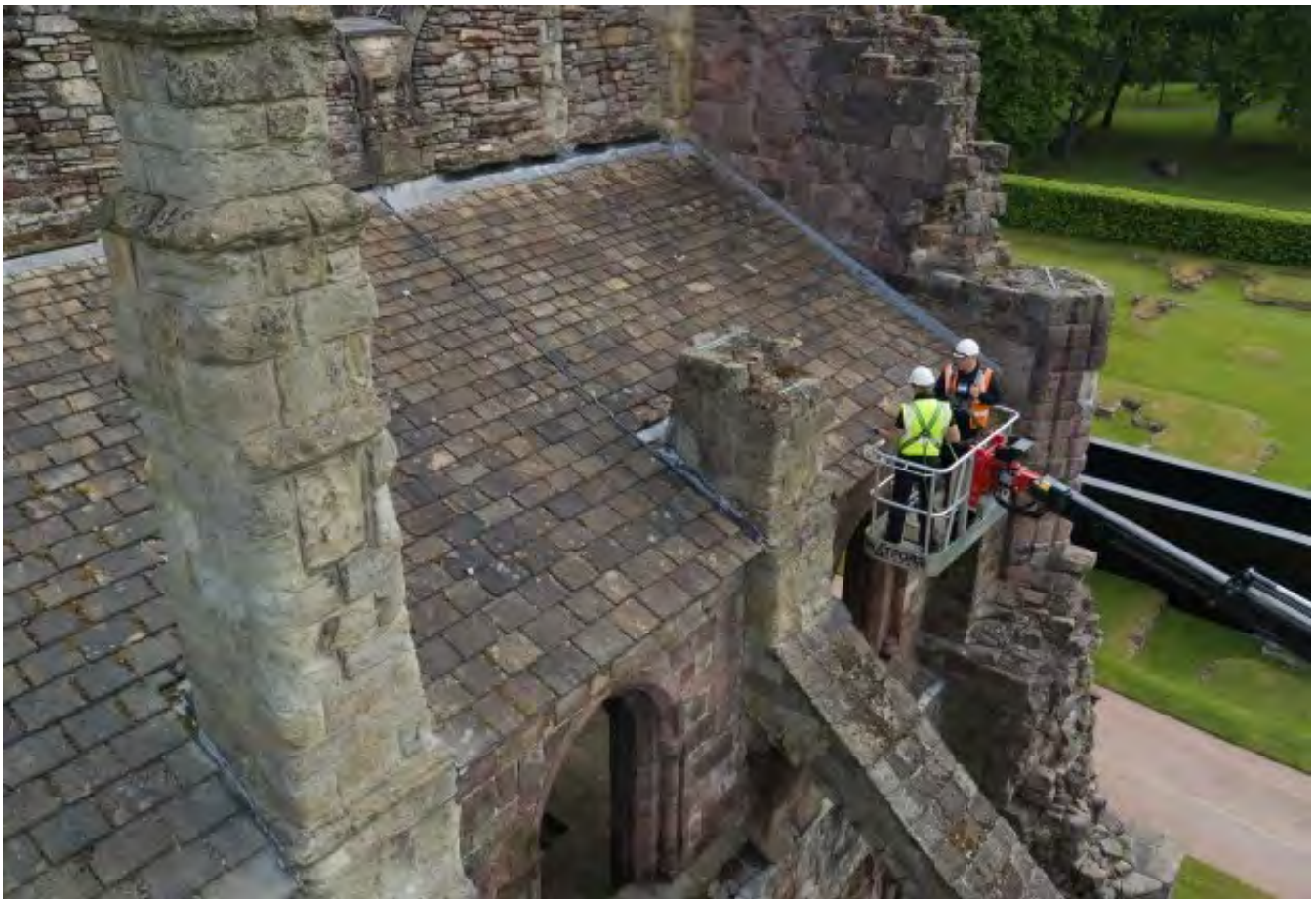
Fig 35. Alexandre, Co-Deputy Team Leader completing High Level Masonry Inspections at Holyrood Abbey.
