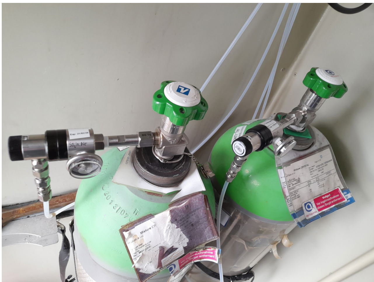
Photo 6: Dial-a-Flow Type Regulator
