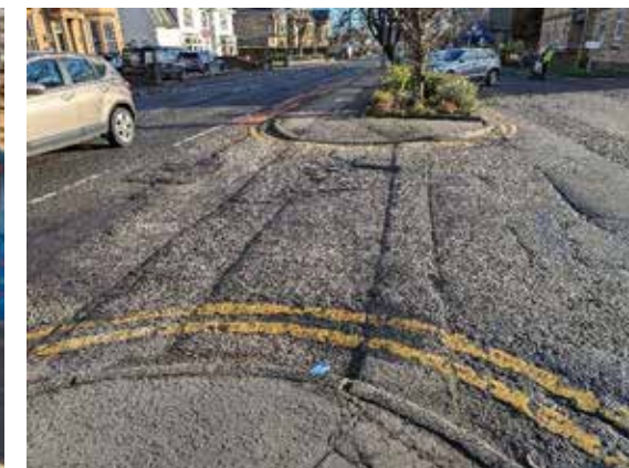
Figure 2-7: Example of dropped kerb access points in poor state of repair
