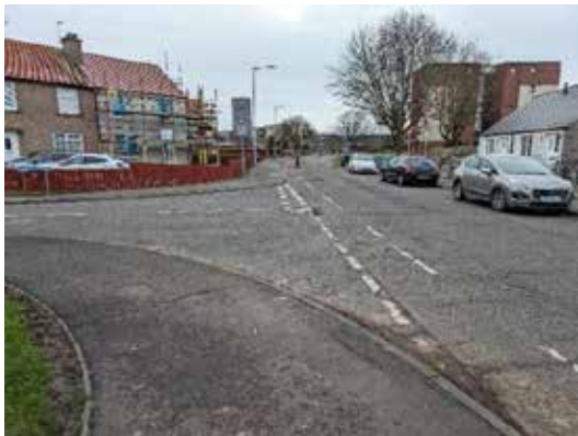
Figure 2-2: Example of lack of dropped kerbs
