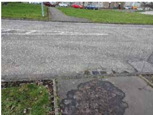
Figure 2-4: Example of lack of dropped kerbs
